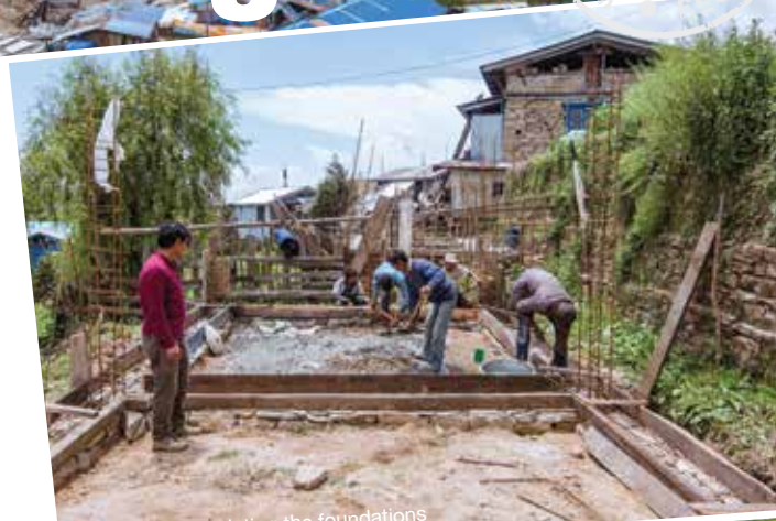
Photo: Completing the foundations
